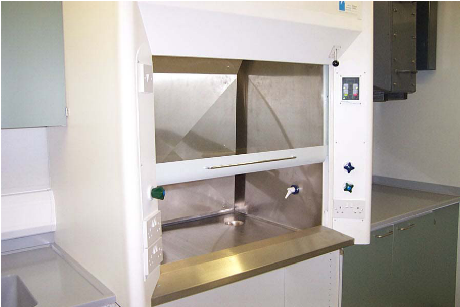
FIG. 9.7. Fume cupboard suitable for use with radioactive materials.
